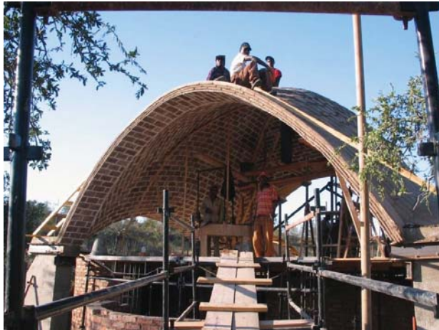
Fig. 2. a) First completed vault of the Mapungubwe project in South Africa (Image credit: James Bellamy); b) Unreinforced thin-tiled floor system of housing prototype for Ethiopia: simple barrel vault with stiffening diaphragms (Image credit: Lara Davis).
