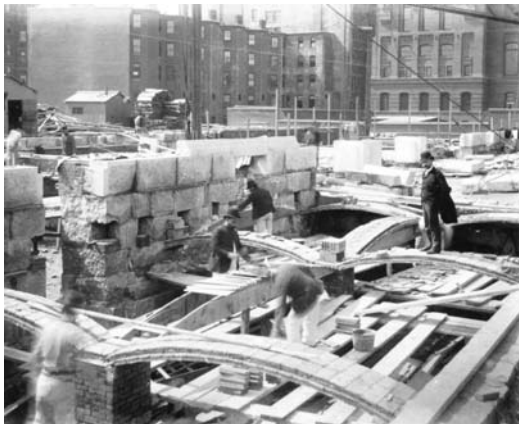
Fig. 3. a) Rafael Guastavino standing on a newly built arch during construction of the Boston Public Library, Boston, Massachusetts, 1889. [10] b) Guastavino Rib and Dome System, New York, 1902. [11]
