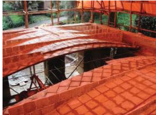
Fig. 2. a) First completed vault of the Mapungubwe project in South Africa (Image credit: James Bellamy); b) Unreinforced thin-tiled floor system of housing prototype for Ethiopia: simple barrel vault with stiffening diaphragms (Image credit: Lara Davis).
