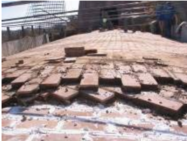
Fig. 4. a) Layered tile construction at Mapungubwe (Credit James Bellamy) b) Tile vaulting, built from multiple layers of thin bricks laid flat [9]
